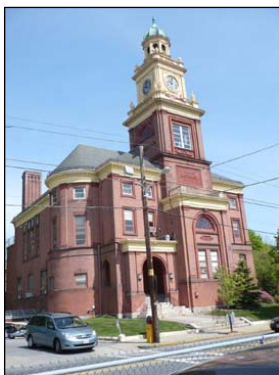
Cumberland Town Hall, 45 Broad Street, Valley Falls
